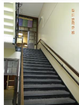
Manufactured stair risers & a custom high-low handrail were incorporated into the stair to make them fun & functional for children using them.
