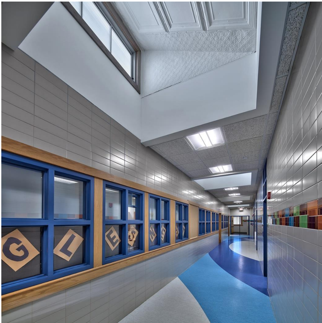
Clerestory windows extend daylight into the corridor on the Second Floor, as well as highlight the re-stored tin ceilings.
