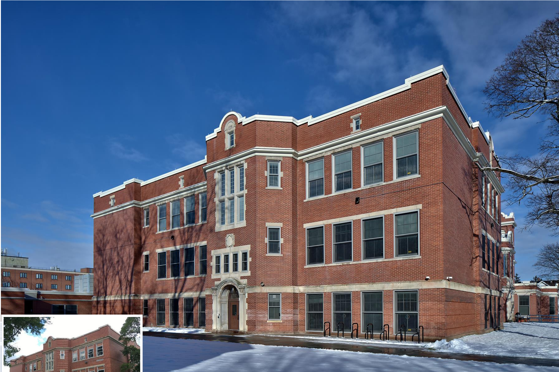
The South portion of the building, which was the original 1910 Schoolhouse, was revitalized. The façade, like many others throughout the building, had the masonry restored, replacement double-hung windows installed & an upgraded entry system.
