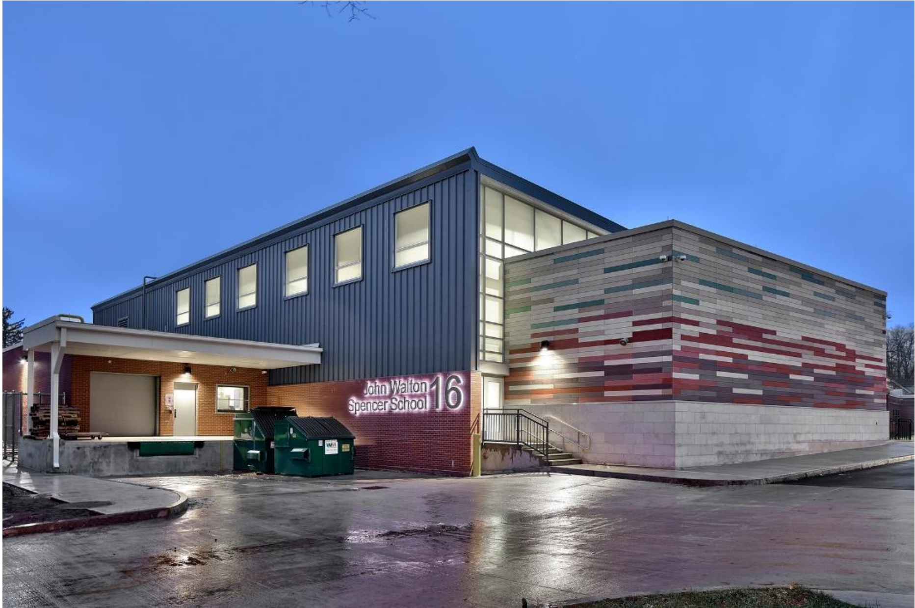
The Gymnasium volume is wrapped in a high-rib insulated metal panel & translucent glass that allows light to penetrate the space without glare, as the Stage façade is activated by a concrete rainscreen system that emulates the motion & energy taking place within the building.
