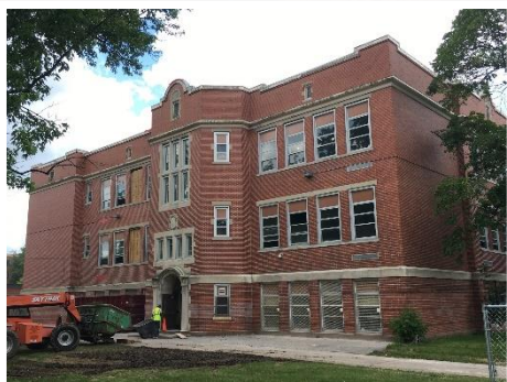
The South portion of the building, which was the original 1910 Schoolhouse, was revitalized. The façade, like many others throughout the building, had the masonry restored, replacement double-hung windows installed & an upgraded entry system.
