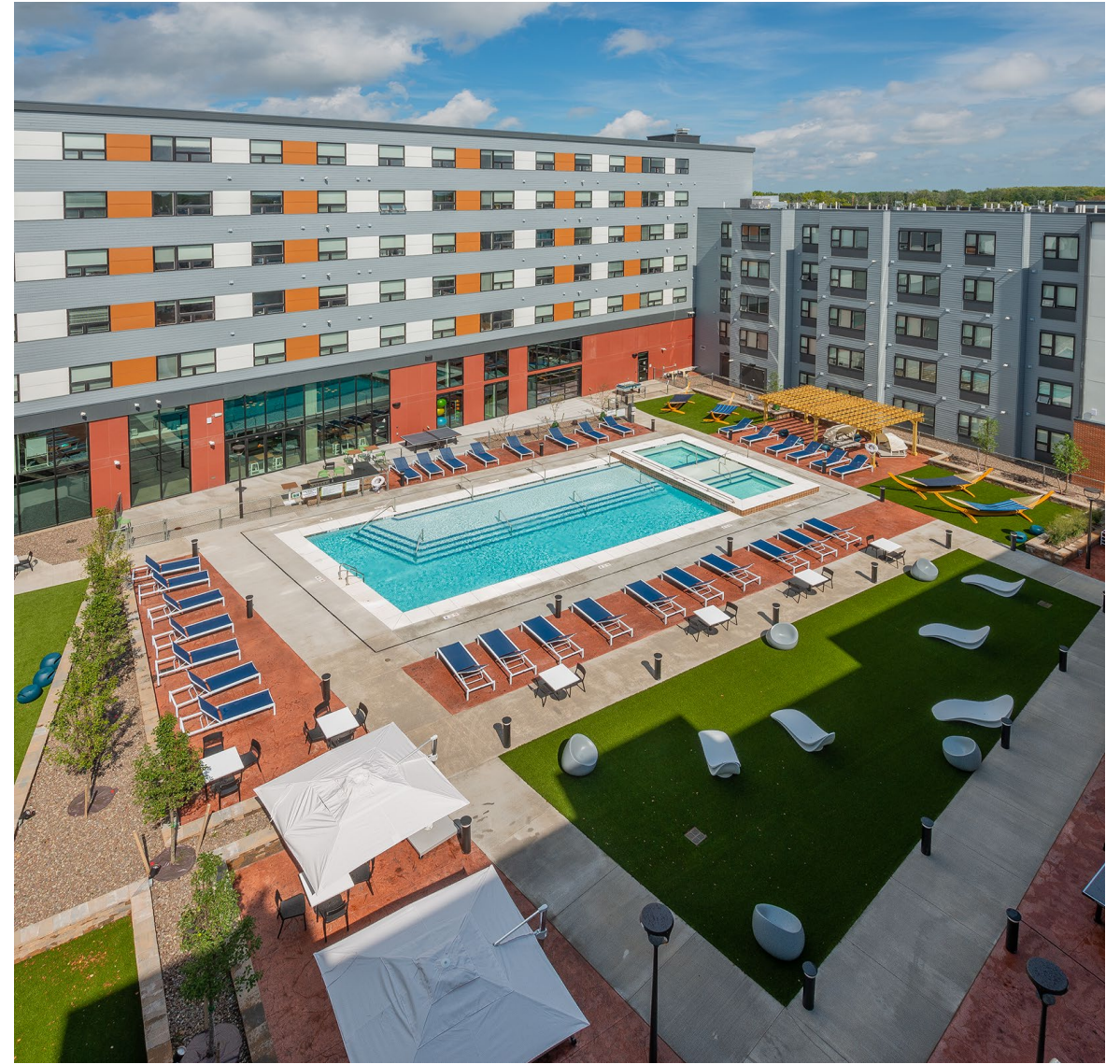
By introducing high density to the site, integration of communal space encourages engagement. The North Courtyard fosters pastimes like barbequing and fire pits while the South Courtyard focuses on sunbathing and relaxing.
