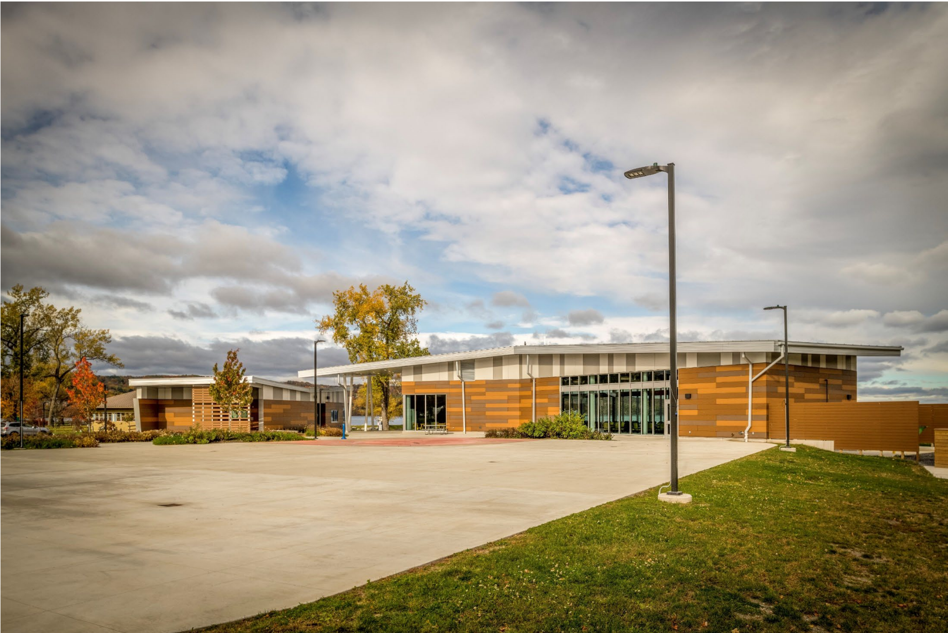
Patio Looking North
