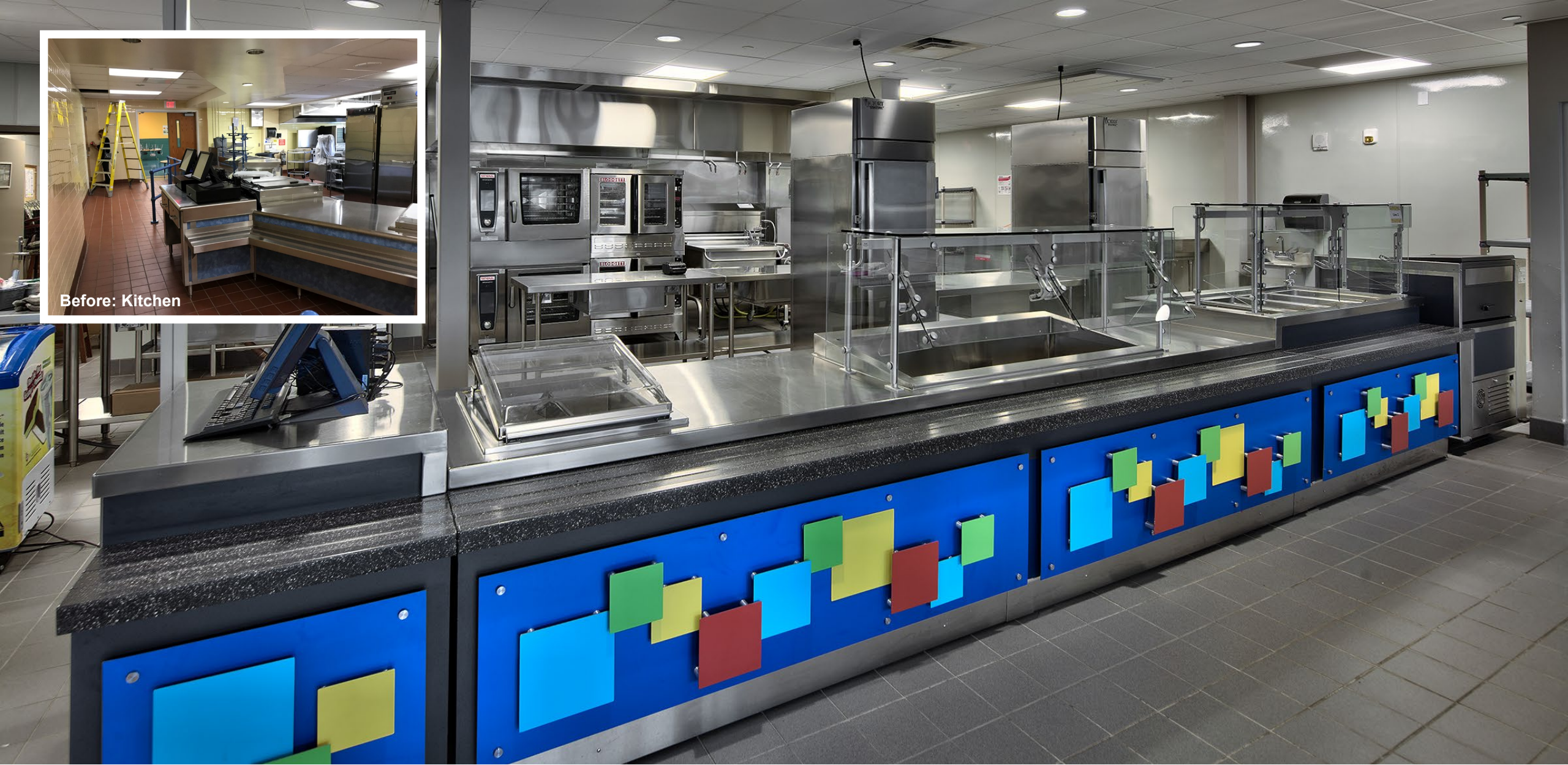
The kitchen footprint has been expanded to twice its original size and has two mirrored serving lines to service the additional student body and is visually connected to the Cafetorium.
