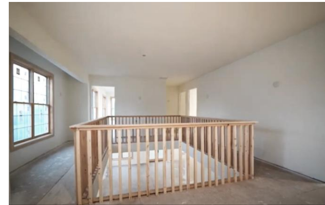
Second Floor Railing Before
