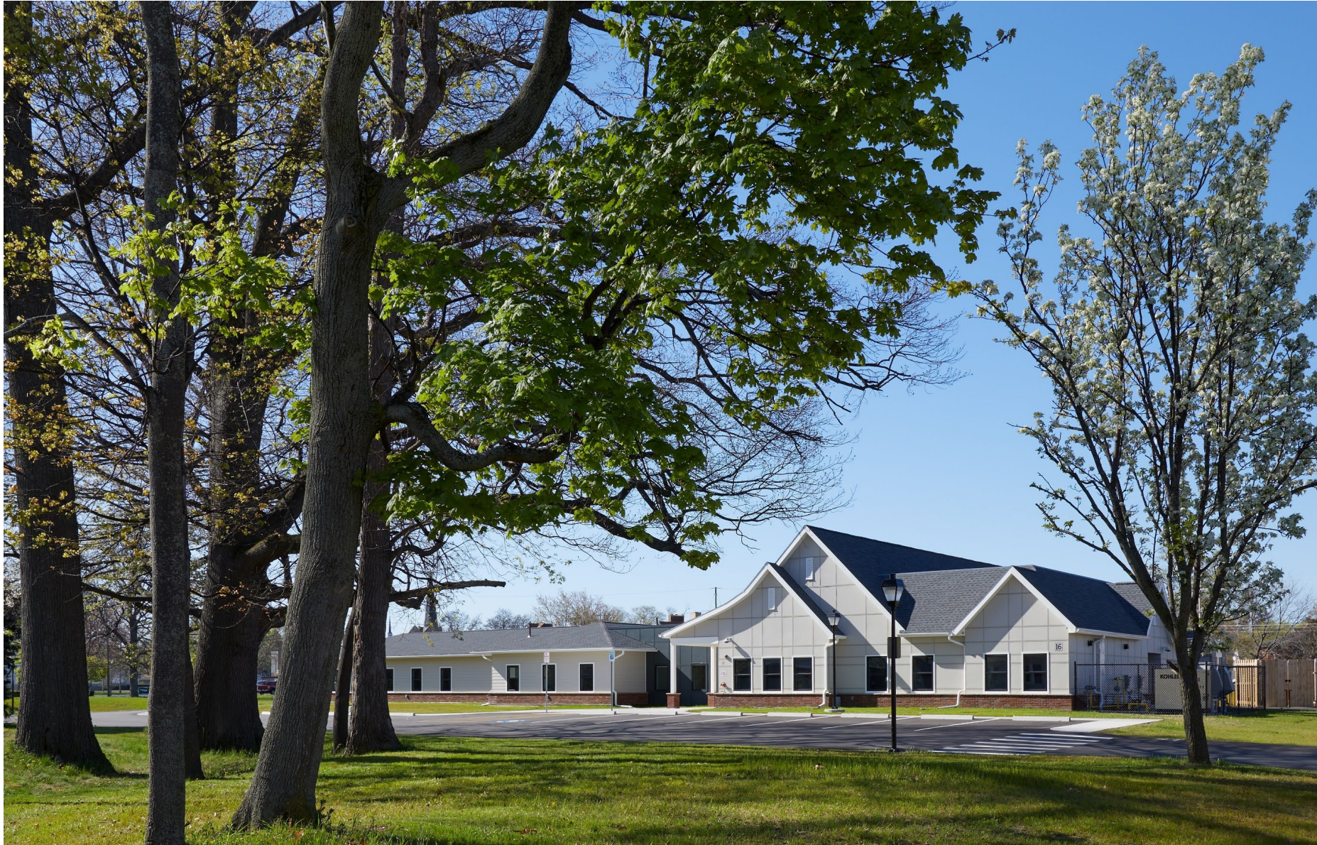
Exterior Photo: Entry Elevation, Facing Villa Campus
